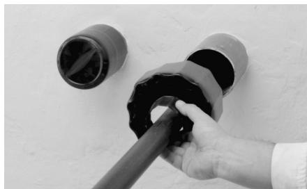
Wipe loose dirt from PVC duct and simply slip LTER or LTCP over the duct.
